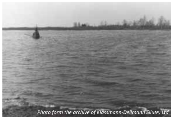
Strong flood waters have destroyed embankments of Aukstumale peatbog (The great flood of 1958). ▼
